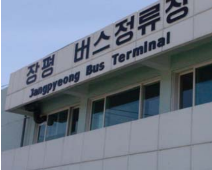
● Jangpyeong Bus Terminal Building
