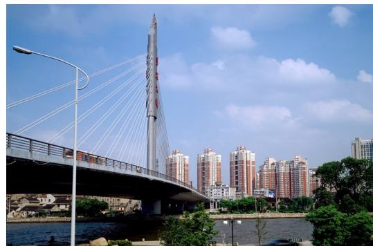
Figure 6. The Ronghu Bridge in Wuxi
