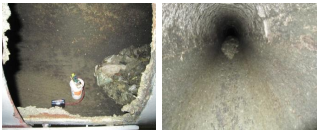
Fig.6. ZigBee communication testing in T-NWK stained horizontal pipe.
