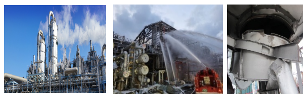
Figure 1. The VOCs emission RTO and gas explosion
