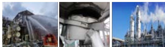
Figure 1. The VOCs emission RTO and gas explosion
